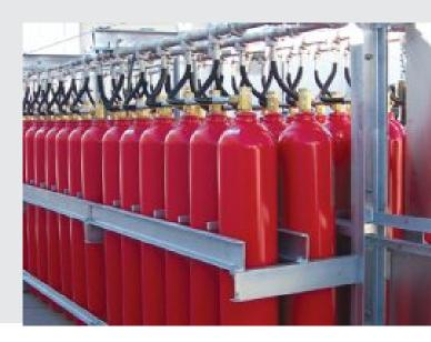
CO2 is the only gaseous agent where the design rules specifically provide guidance on the protection of deep seated hazards.
